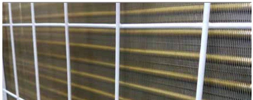
Golden Fin: anti-corrosion protection on the exchanger
